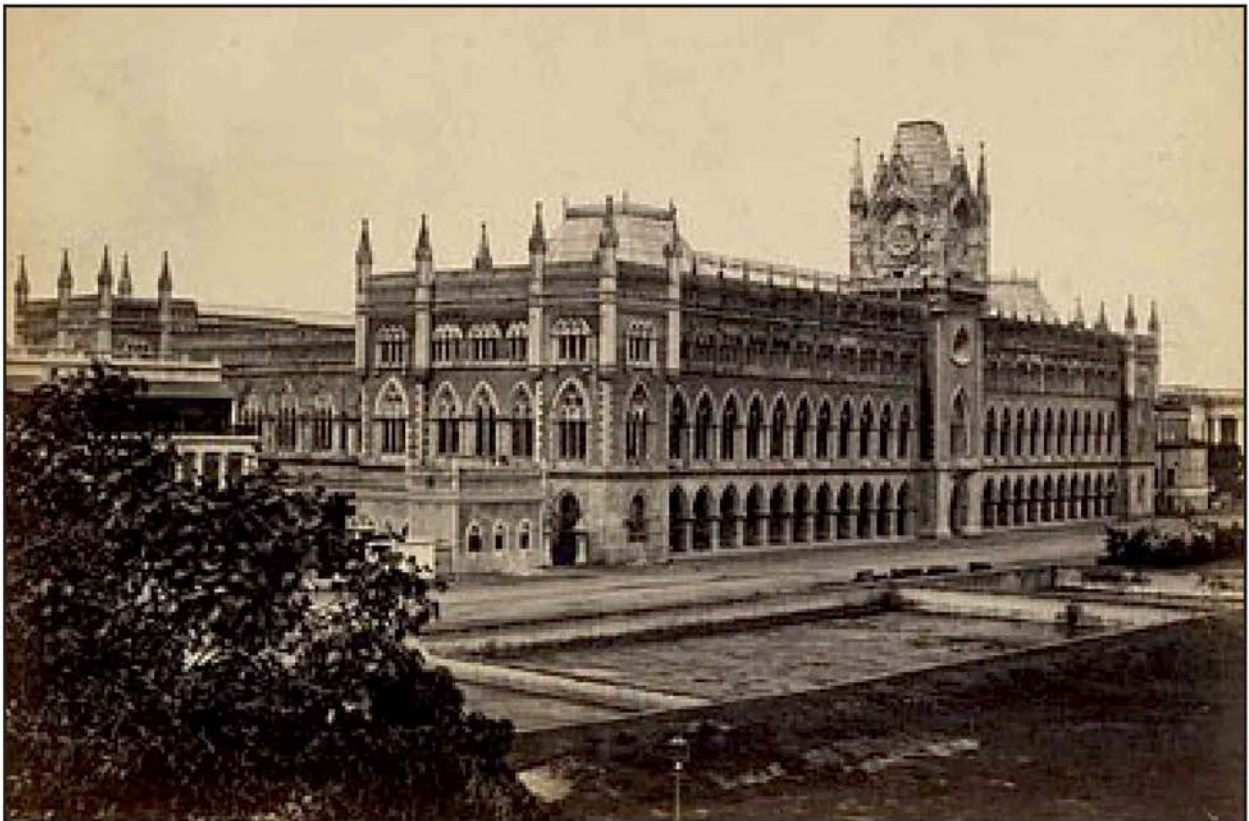
The High Court at Calcutta nearing completion
