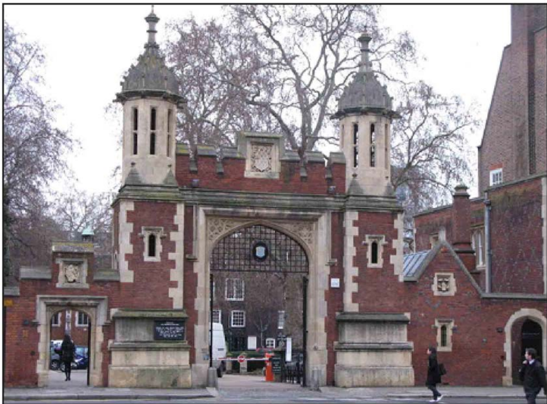
The Gate House
