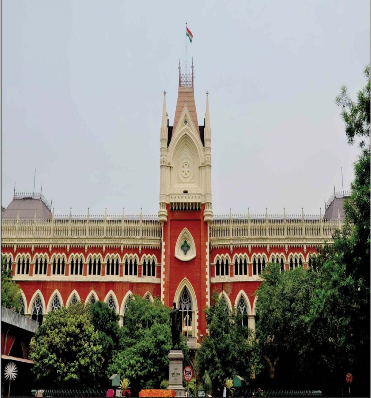
The Main Building of the High Court at Calcutta
